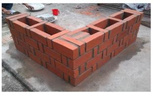
Fig.1 Typical picture of Rat-Trap bond
