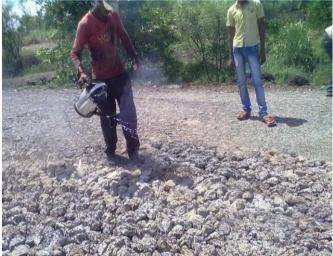
Fig. no.3- Bitumen spreading
